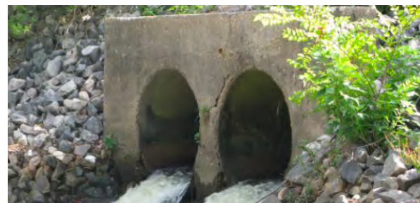
Combined sewer outfall. Photo credit: Gary Green Infrastructure Plan (2019)
