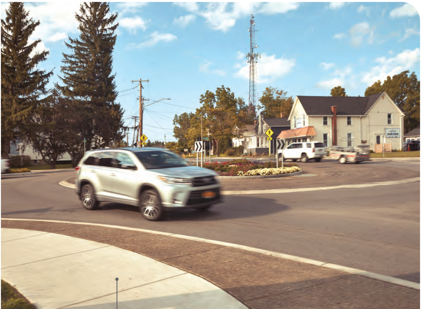
Traffic signals were replaced with two landscaped roundabouts in the Village of Lancaster as part of its West Main Street Extension Project. The slower but safer and more efficient flow of traffic has led to a reduction in emissions and intersection delays.
