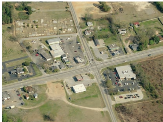
Historic hamlets like Hephzibah grew at a time when the ability to walk between commerce and residences was important
