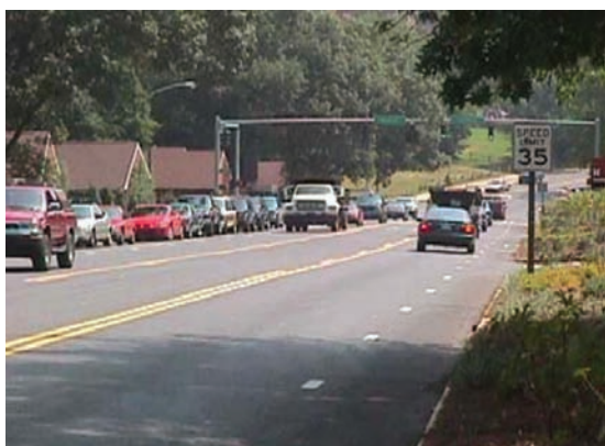
Same stretch of roadway, after their "road diet" reduced crash frequency along the corridor by 53% while creating a designated bike lane and increased roadway plantings.
