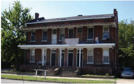
15th Street, originally worker housing
