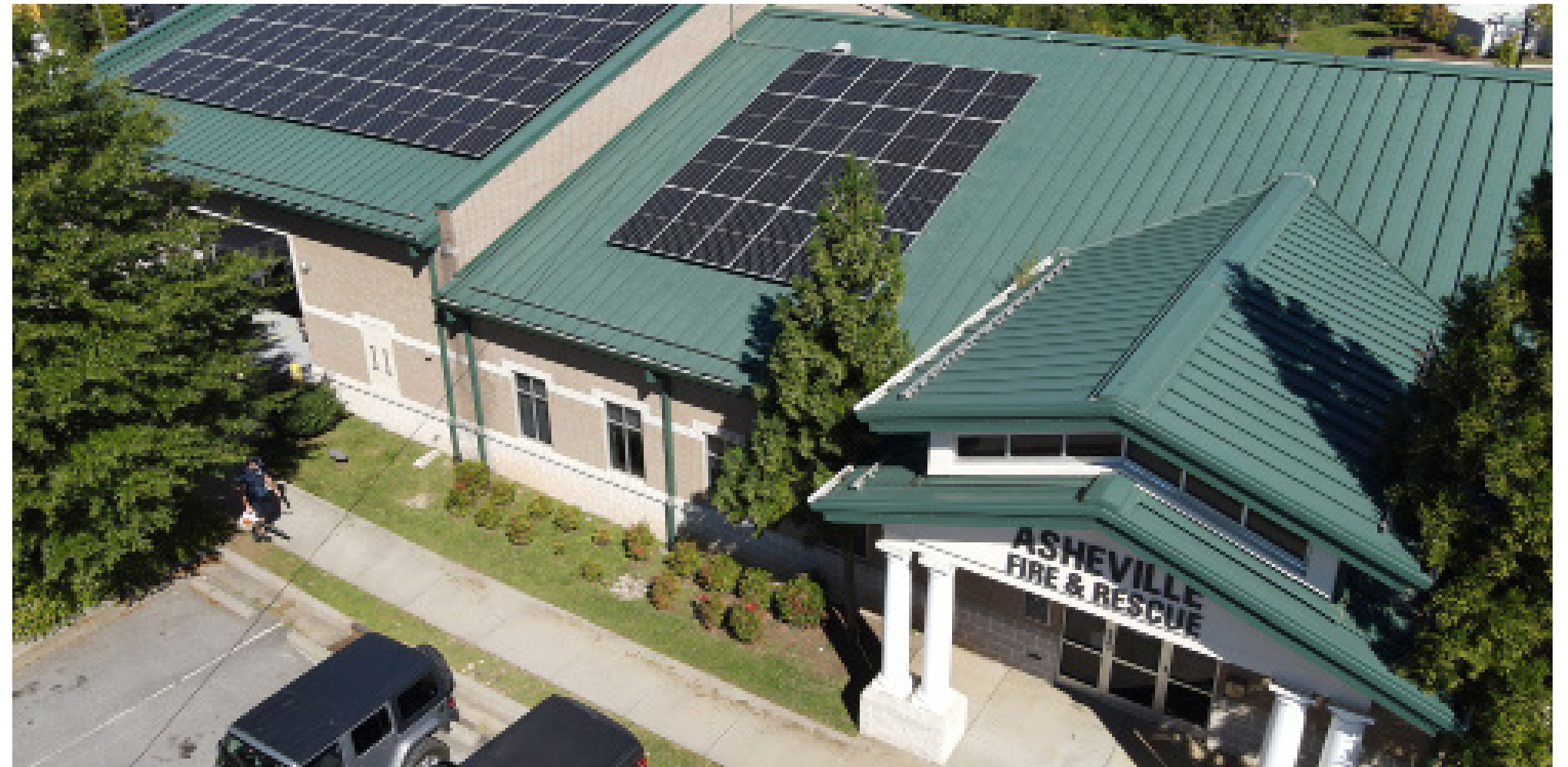
Solar Array at Fire Station #11
