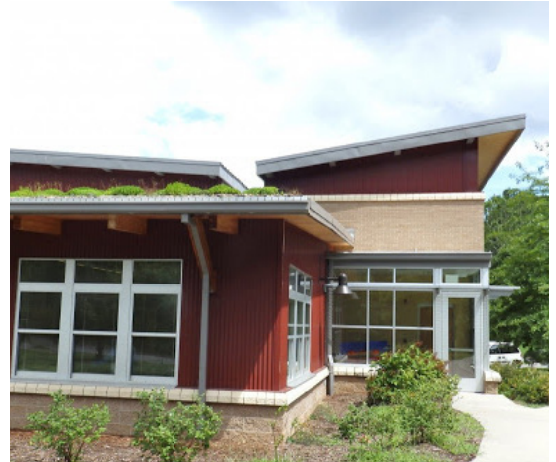
Green roof at the Dr. Wesley Grant Sr. Southside Community Center
