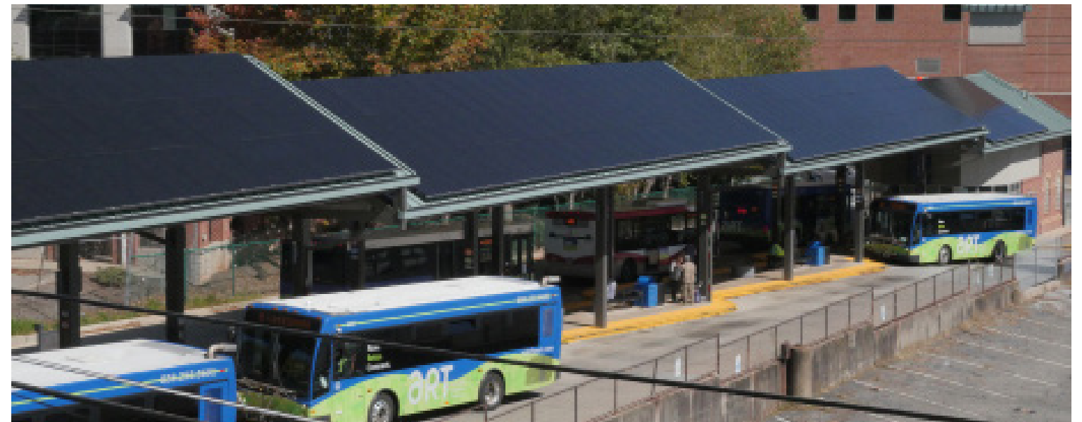
57.4 kW Solar Array at the ART Transit Center
