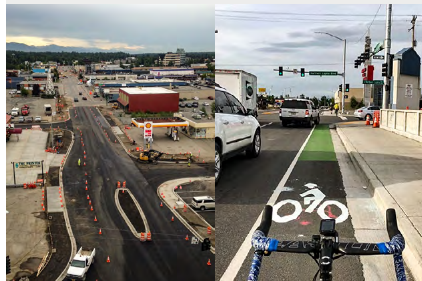
The first Complete Streets project in Anchorage was for Spenard Road, and featured colored bike lanes, wider sidewalks, and improved pedestrian crossings. Photo credit: Charles Boyle (left) and Brian Looney (right)
