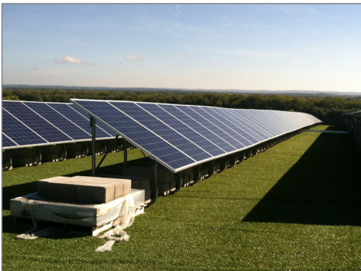
Hartford has a 1 MW solar array on top of its now-capped landfill in the North Meadows, which saves taxpayers money while repurposing an environmental liability.
