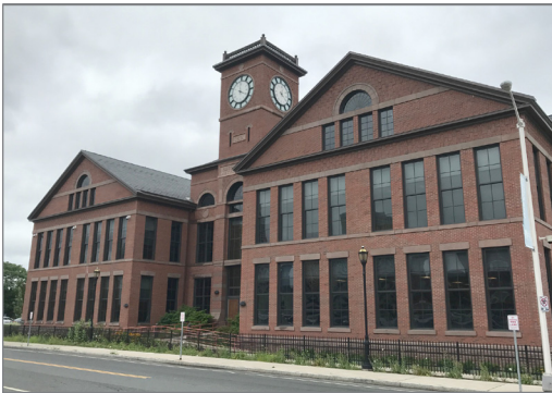
The Public Safety Complex, which houses police and fire headquarters, has saved 10% in energy reductions from the baseline year in 2014, due in part to retrocommissioning and efficiency suggestions from a third party partner.
