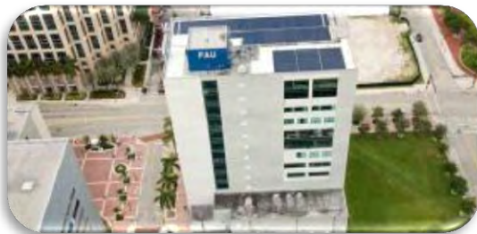
Pictures: FAU’s downtown campus solar system and real-time monitor
