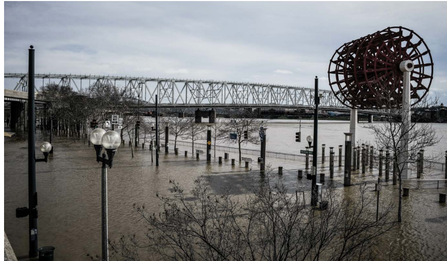
Flooding caused by severe storms.
