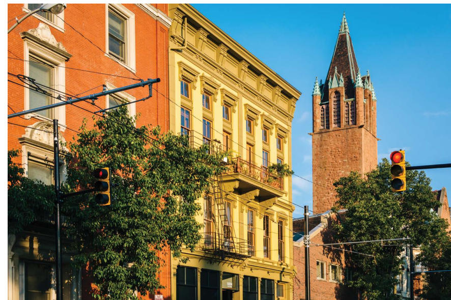
Cincinnati has an older building stock that can benefit from energy efficiency upgrades.
