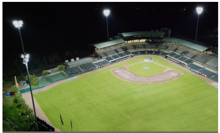
New LED lights at Joseph P. Riley, Jr. Ballpark.
