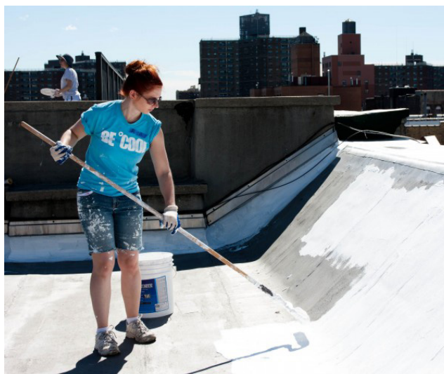
2.6 million square feet of roofs in New York City have received a "Cool Roof" coating. (Photo by Tara McIsaac, Epoch Times.)
