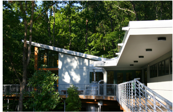
Ruffner Mountain's Treetop Visitors Center earned a LEED Gold designation in 2011. The center's green design features include stormwater recycling, a green roof, energy efficient lighting and control systems, and use of recycled and locally-produced building materials. (Photo: KPS Group, Inc.)
