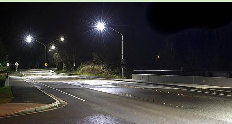
Before (above) and after (below) LED streetlight installation
