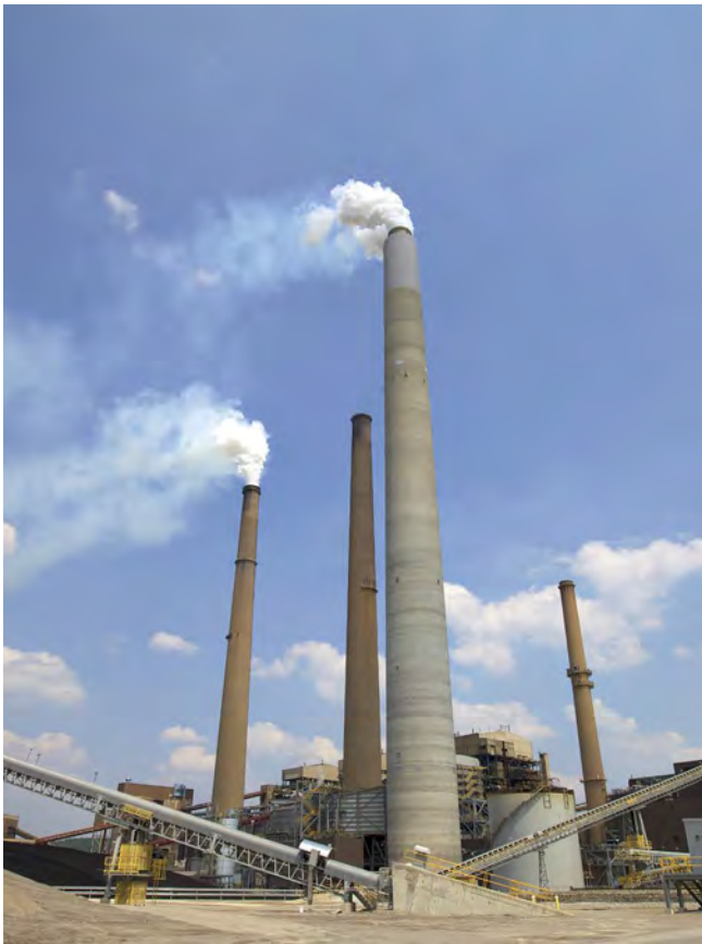
Conesville Plant in Coshocton County, Ohio, which opened in 1957, retired from commercial operation in May 2020. Through most of its life, the coal-fueled generating facility operated six units.
