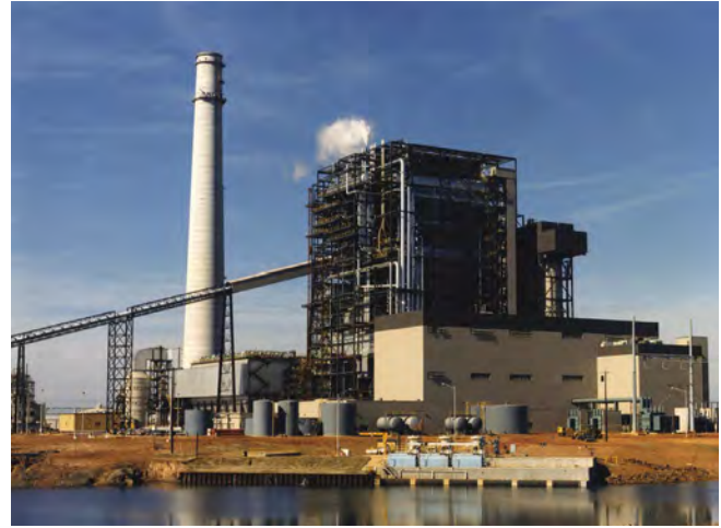
Pirkey Plant will retire from commercial operation in 2023.
