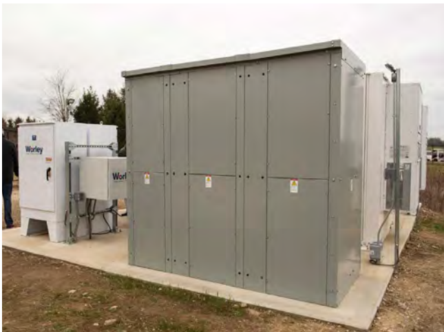
The 138 kilowatt solar panels and pair of batteries (pictured) will help the zoo cut energy costs and reduce its carbon footprint.
