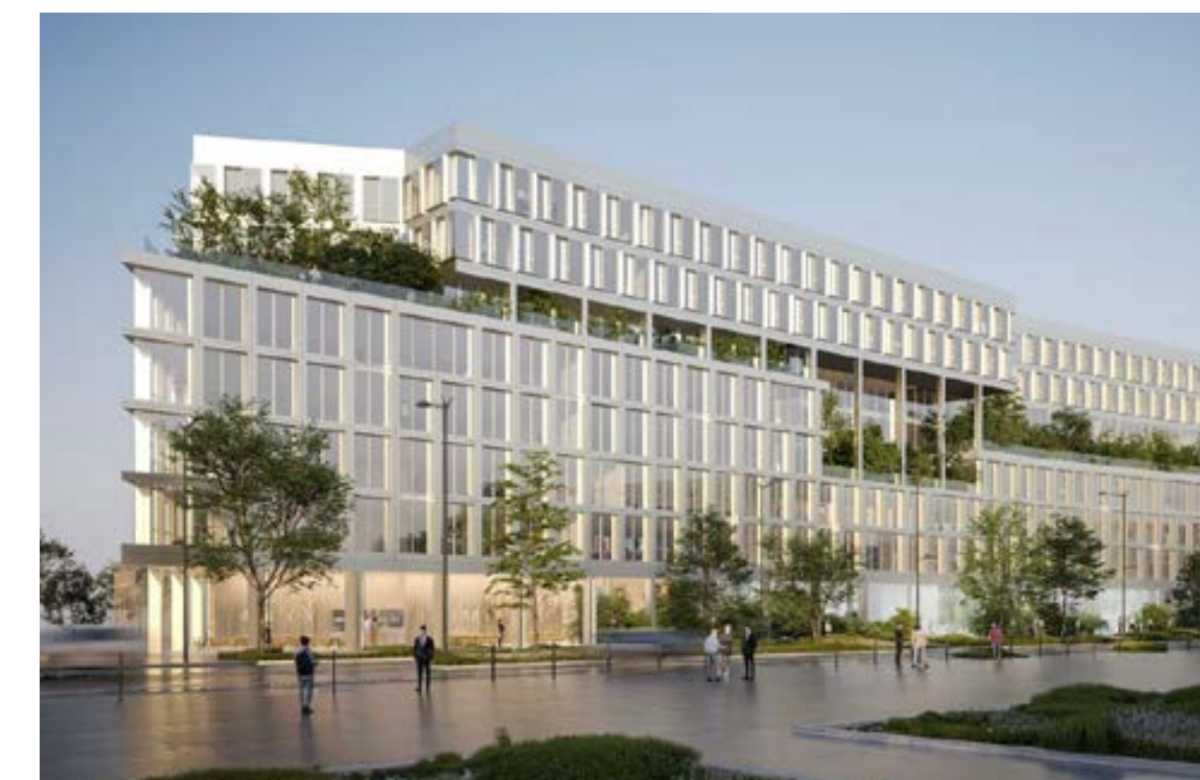
This building owned by Allianz has the following certifications: Label Effinergie BBC 2017, BiodiverCity and HQE New Excellent.
